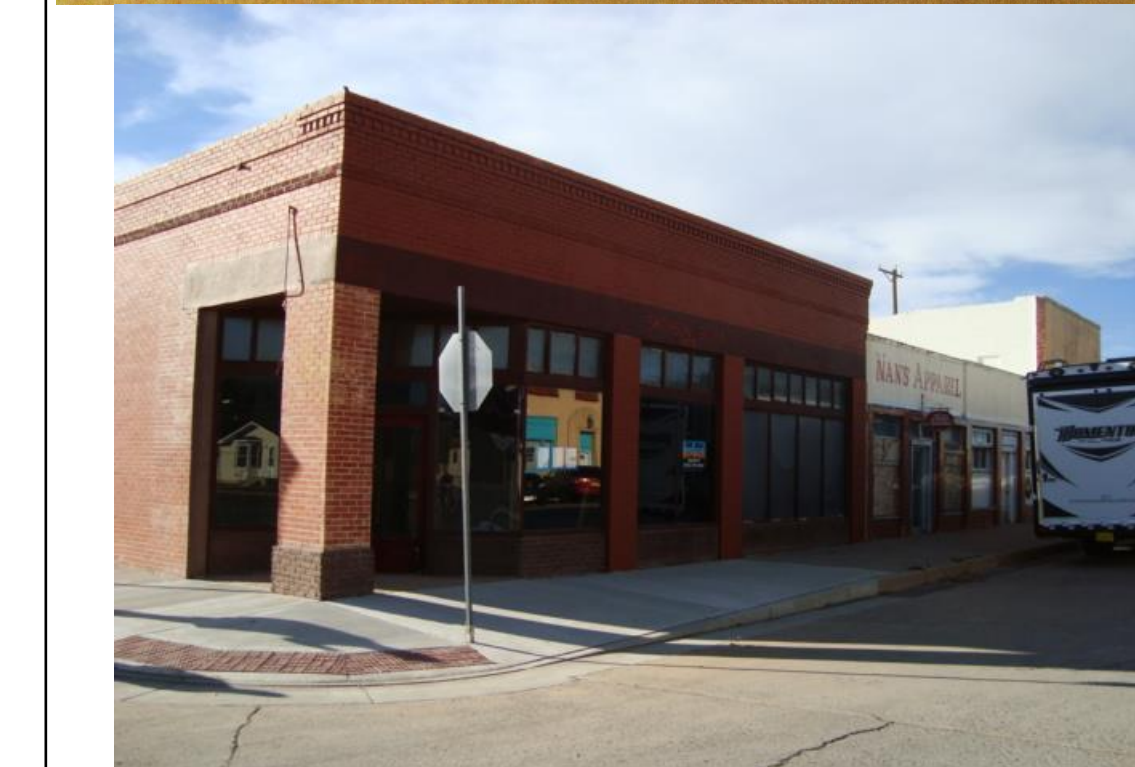
Brane Mercantile, looking Southwest: Historical (Top) & Present day (Bottom)
